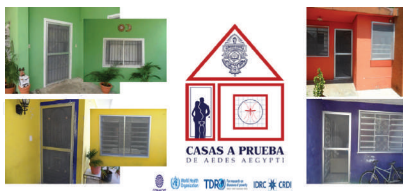
Figure 1. Photographs show Aedes aegypti -proof houses with insecticide-treated screens mounted on aluminium frames and fixed to external doors and windows of treated houses.
